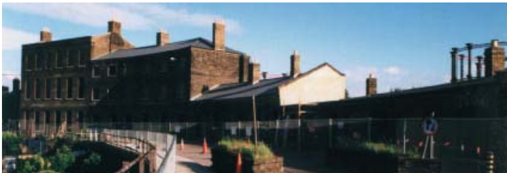
Figure 3: Coal and Fish Buildings under repair. Author photograph.
