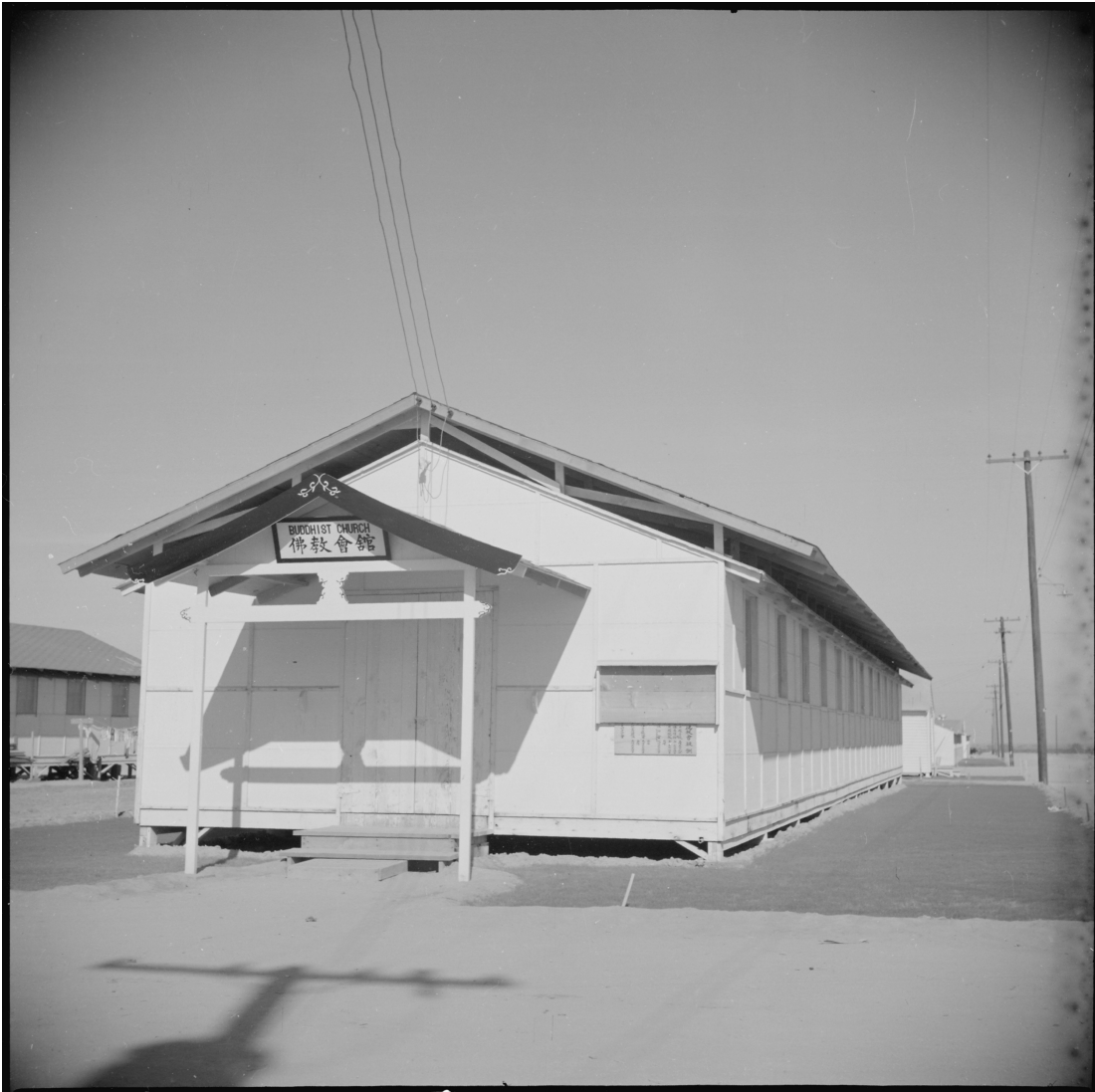
Figure 3. “Gila River Relocation Center, Rivers, Arizona. The Buddhist Church at camp two at this relocation center” (Francis Stewart, WRA Photographer, November 27, 1942) https://catalog.archives.gov/id/538609
