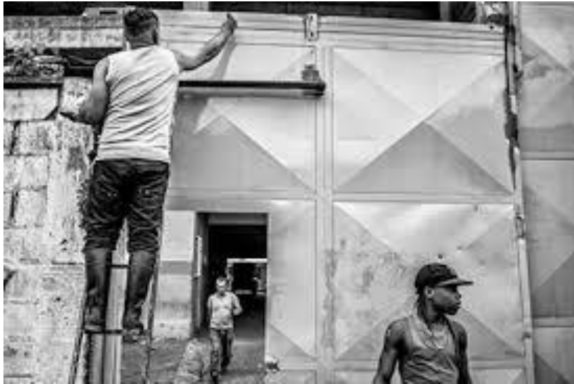
Figure 6: Resident working on construction in Torre David. Alejandro Cegarra, 2012.
