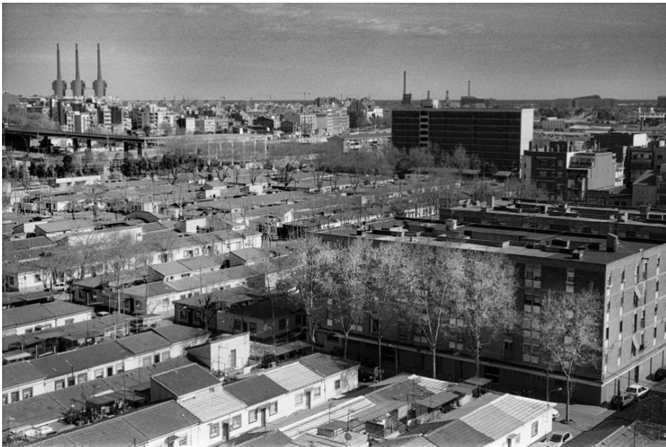
Figure 1: Bon Pastor before the demolitions (Carola Pagani, 2005)
