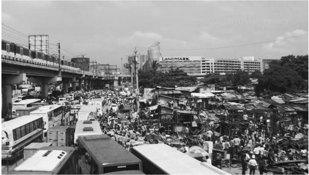
Figure 4: A 2010 picture of the demolition in the EDSA part of Sitio San Roque. Photo is from Ilang Ilang Quijano.
