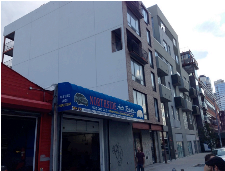
Image 11: Auto repair shop next to a long row of luxury condos that extend to the East River waterfront (Williamsburg)
